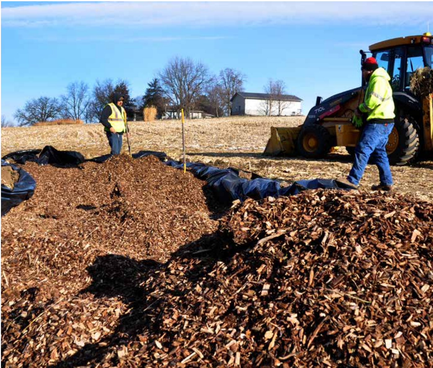
▲ The installation of a wood chip bioreactor. Wood chips remove nitrates from tile water as the water flows through the bioreactor. © SWCS/IDALS Photo by Lynn Betts
