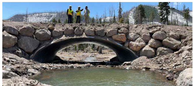
Figure 3: Completed bottomless arch culvert with locally sourced stone applied to headwalls and stream grade control. Construction efforts are later supplemented with the planting flood resilient vegetation, such as willows, to reduce erosion, increase bank stability and restore habitat for fish and wildlife. Credit: Dave Turk, AECOM
