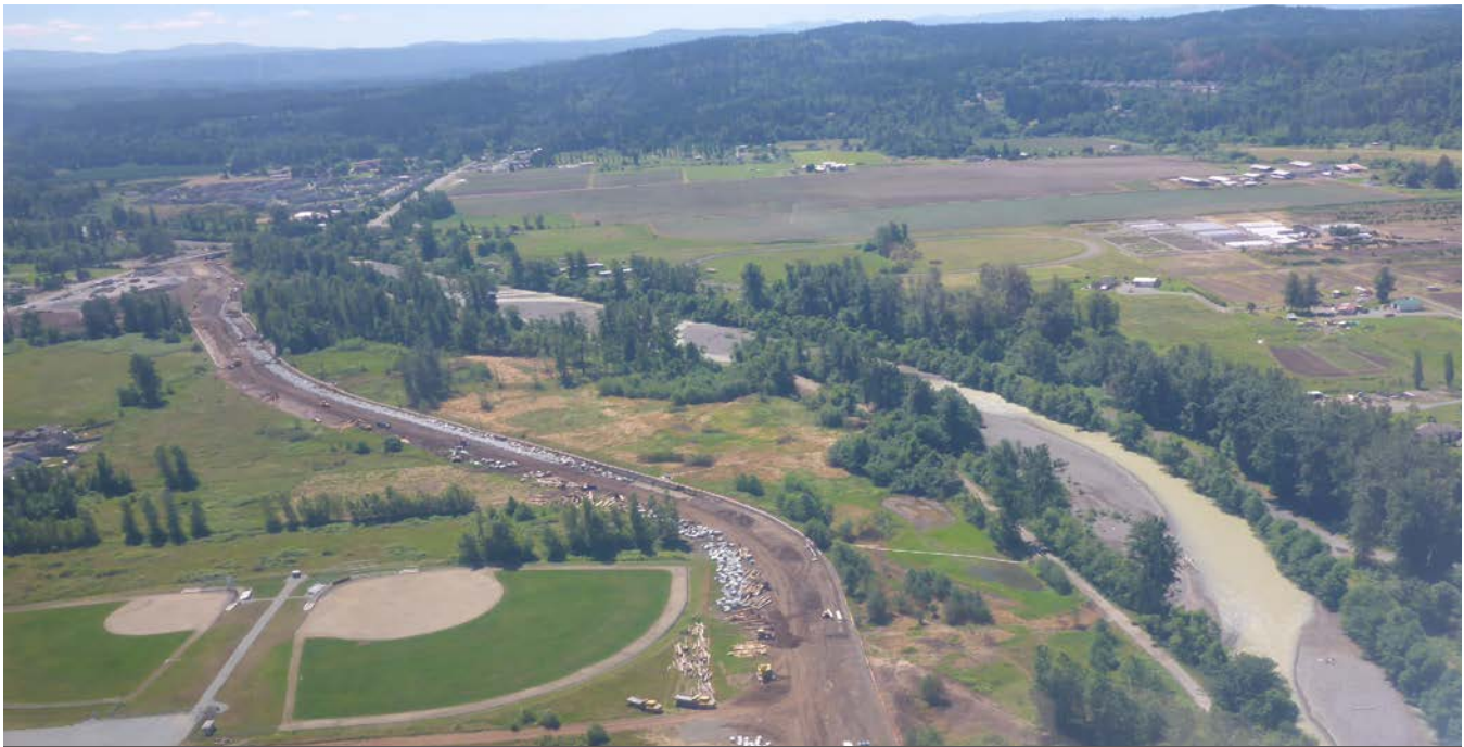
Figure 1: Calistoga Reach Levee Setback. Credit: City of Orting. 10
