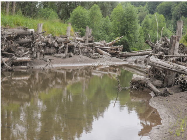
Figure 2: Engineered logjams on the Puyallup to generate suitable salmonid habitat. Credit: The Nature Conservancy 5
